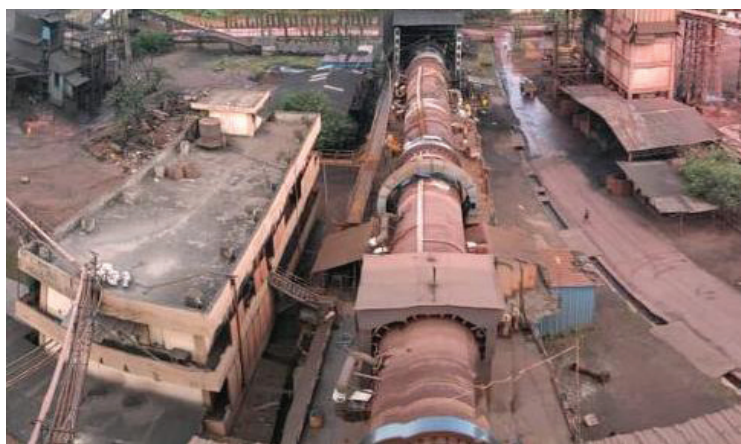
Figure 14: Pictorial view of rotary kiln in DRI plant
